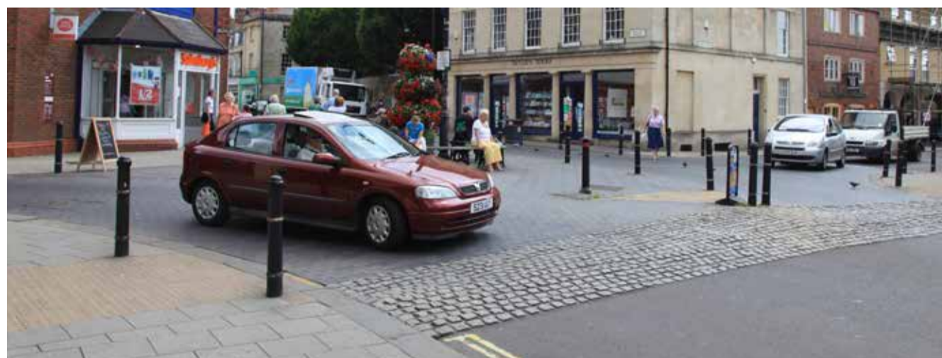
Raised junction, change in carriageway material and use of vertical elements
